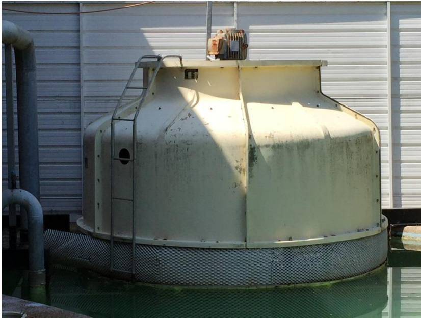
BUDGE ELLIS COOLING TOWER - type FRP100RT, 100 ton capacity,
