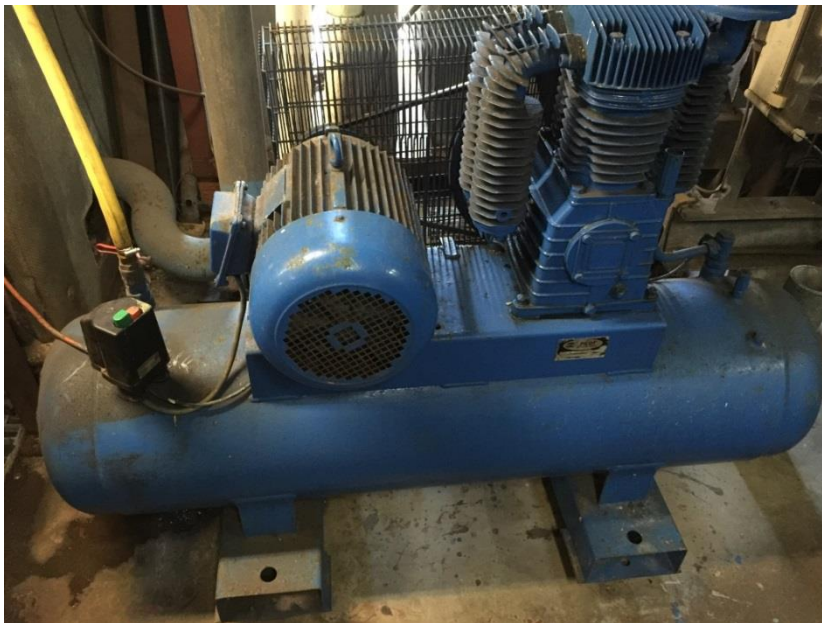
K30 PILOT AIR COMPRESSOR
